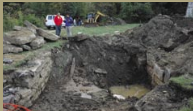
In the fall of 2006, archaeological investigations showed that the stone walls of Lock 2 East are still intact below ground level.
